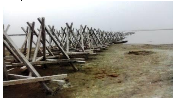
Fig 1: RCC Porcupines laid in Majuli, Assam
