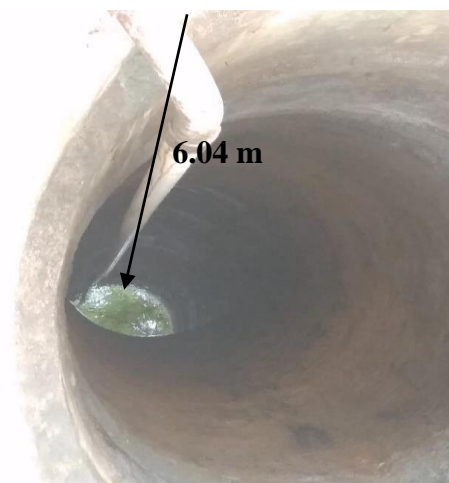
Fig. 1. Well depth in Anandanagar hill slope, Guwahati
