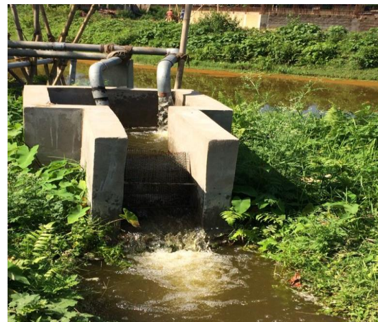
Fig 4: The collecting chamber that receives the water from the pump
