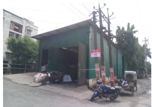
Fig. 1. Secondary Transfer Station at Zoo Road
