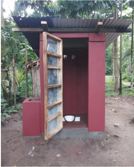
Fig. 5. Construction of IHHLs in Lakhimpur district.
