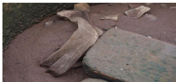
Fig. 2. Reddish layer formed on top of the filter media of the selected filter unit.
